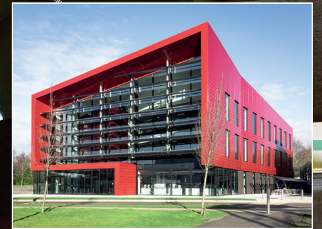
WMG Degree Apprenticeship Centre
